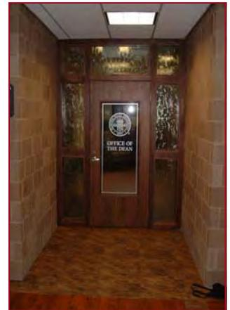
In this two hour wall application, a glazing unit combining fire and decorative glass was used in the transom and sidelights, along with custom trim on the frame. The wood door was fitted with vision light kit and clear glazing
