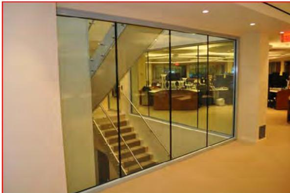
Interior one hour butt-glazed system utilizing Aluflam framing system. Glazing is Contraflam Structure 60 by VSGNA.
