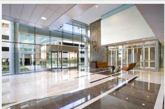
Application of open concept meeting Code with fire rated curtain wall at exterior and interior system at vestibule.
