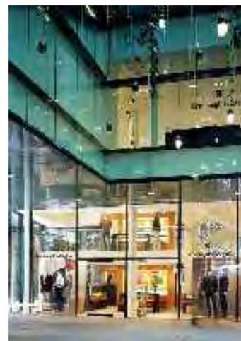
One hour fire rated, butt glazed wall system by Vetrotech Saint-Gobain. Includes entry door option.
